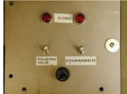
Figure 4 – Panel holding the roughing switches
